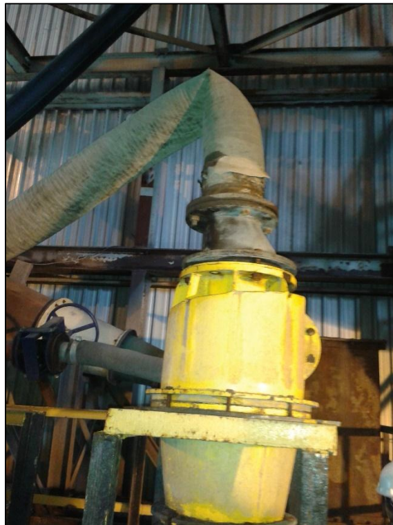
Figure 18: Flexible hose blocking free flow of material.
